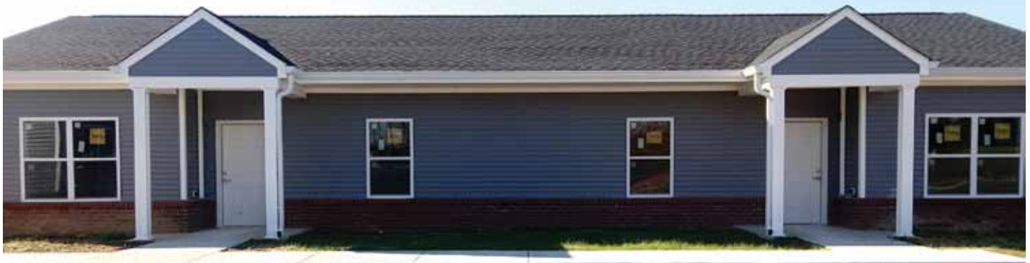
A newly constructed duplex at Jackson Court in Salem will provide affordable housing for people 55 or older and those with disabilities.
